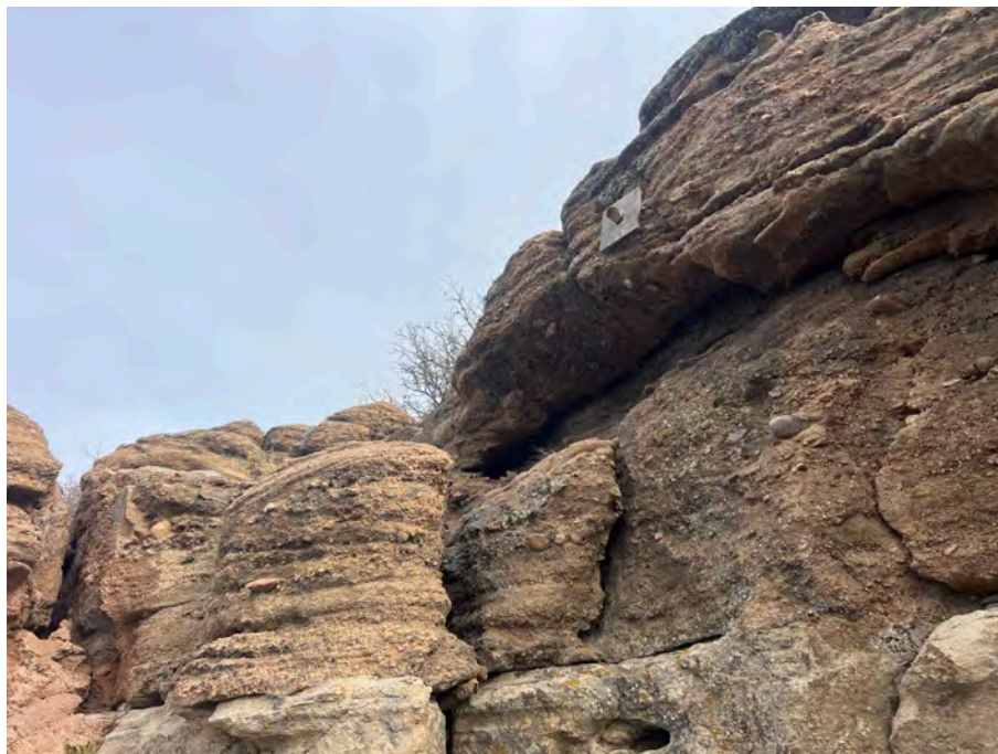
Area 3 West: Rock Bolted Block From Below
